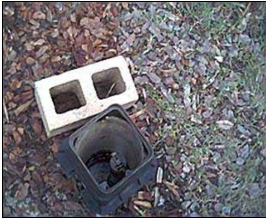
Fuel Storage Tank Filling Point Pelican Boat Hire
