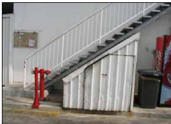
Cabinet for Mobile Fuel Pump De-Brett's Wharf
