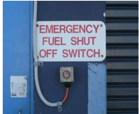
Close up of Fuel Shut-off Location Tabuka Wharf
