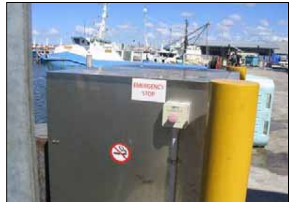
Fuel Pump Emergency Shut-off Mooloolah River Fisheries
