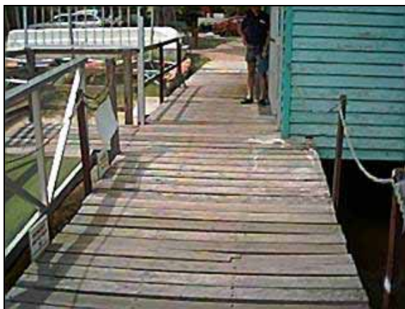
Emergency Shut-off Valve to Left ‘O’ Boats
