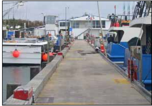
Wharf with 6 Remote Fuel Outlets De-Brett's Wharf
