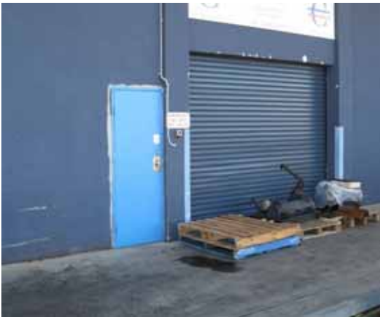
Fuel Shut-off Location Tabuka Wharf
