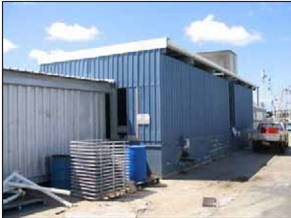
55,000 Litre Fuel Storage in Shed Browns Main Wharf
