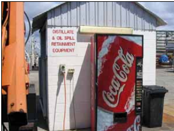
Oil Spill Equipment in Shed Browns Main Wharf
