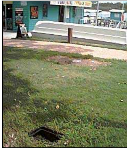
Underground Fuel Storage Tank Filling Point ‘O’ Boats
