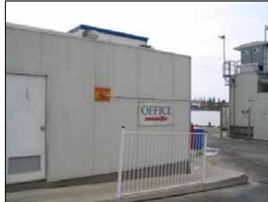
Fuel Pump Emergency Shut-off De-Brett's Wharf
